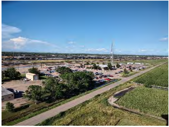
Main office and operations building.
