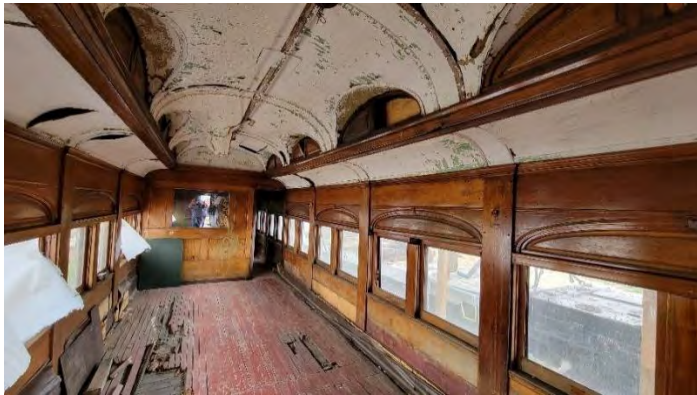
Interior of 1905 Passenger Car
