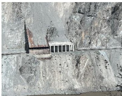
Snow shed and rockslide.
